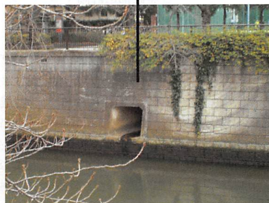
排水渠 (W1.8m × H1.8m)
